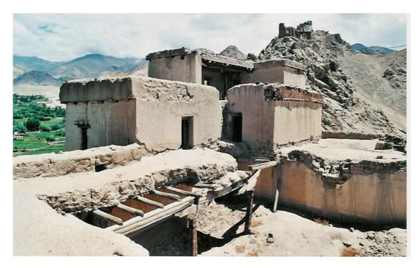
Fig.3. The roof of the Leh palace before its repair by the Archaeological Survey.
